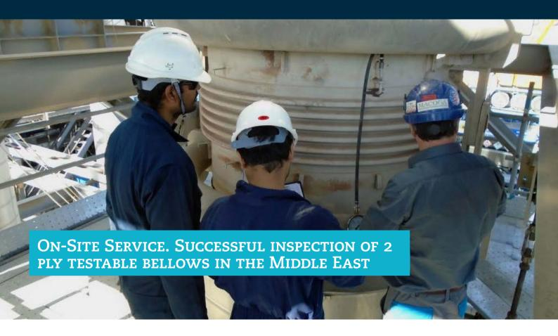
In two ply testable bellows each ply is designed for the full operating conditions (pressure, temperature and movements). If a hole or stress crack develops in the inner ply during service, the outer ply takes over without exposing operators to increased risk or creating the need for an unscheduled shutdown.
